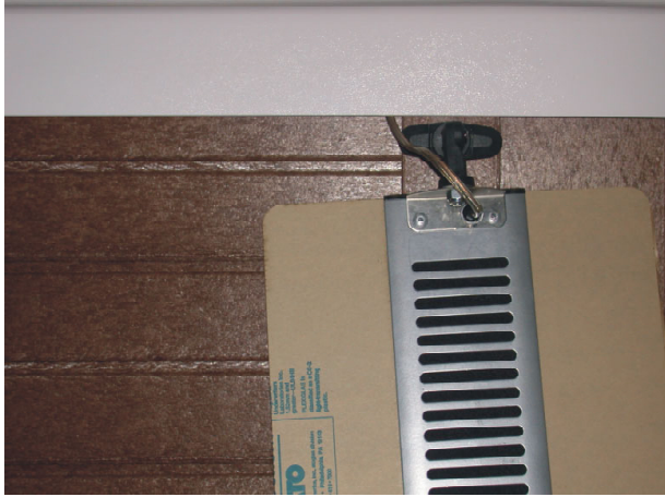
Figure 50. Completed Speaker Installation
